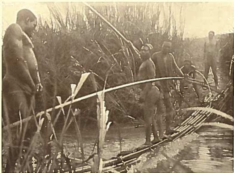
Building a temporary bridge between Kabri and Titong.
